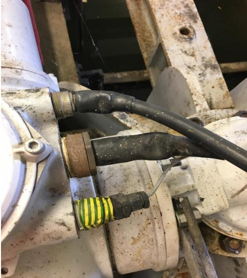
Figure 36: Actuator No.2 cable glands
