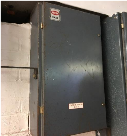
Figure 32: Corrosion on electrical distribution panels
