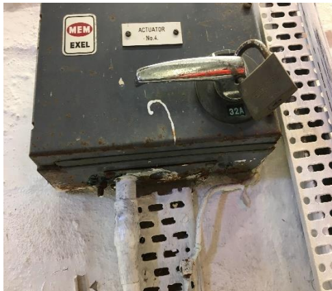
Figure 35: Corrosion on actuators isolators
