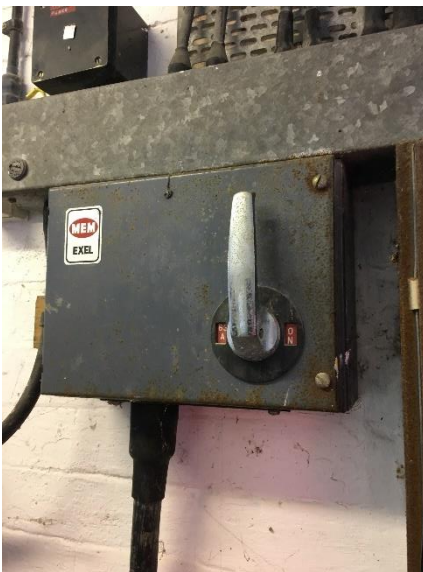
Figure 43: Corroded local isolator
