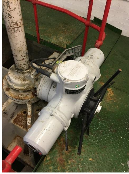
Figure 37: Actuator No.1 with cable glands
