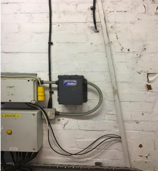
Figure 47: Unsupported cables
