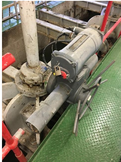
Figure 21: Actuator four – main sluice gate four
