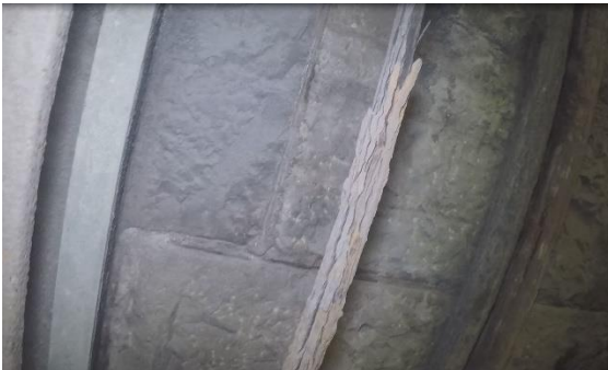
Figure 16: Severely corroded pole – main sluice gate four
