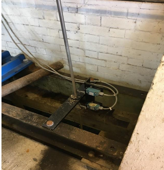
Figure 46: Limit switch cabling
