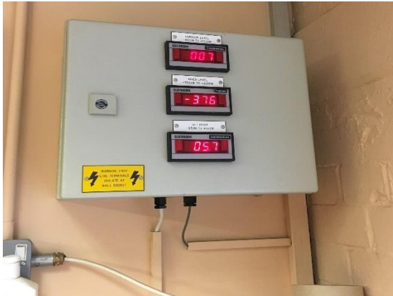
Figure 24: Levels display panel
