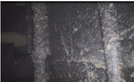
Figure 12: Corrosion on redundant poles– main sluice gate 3
