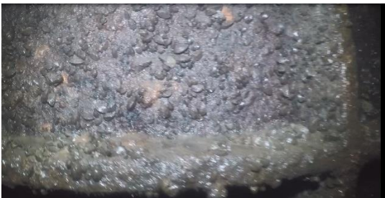
Figure 6: Corrosion and zebra mussels - main sluice gate 1
