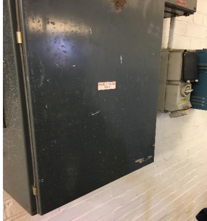
Figure 33: Corrosion on electrical distribution panels
