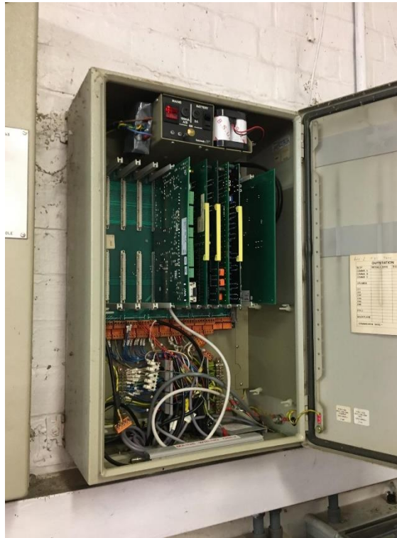
Figure 31: Telemetry marshalling panel
