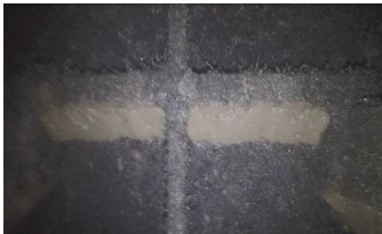
Figure 13: Siltation on gate – main sluice gate 3
