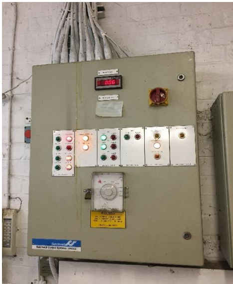
Figure 28: Main sluices main control panel
