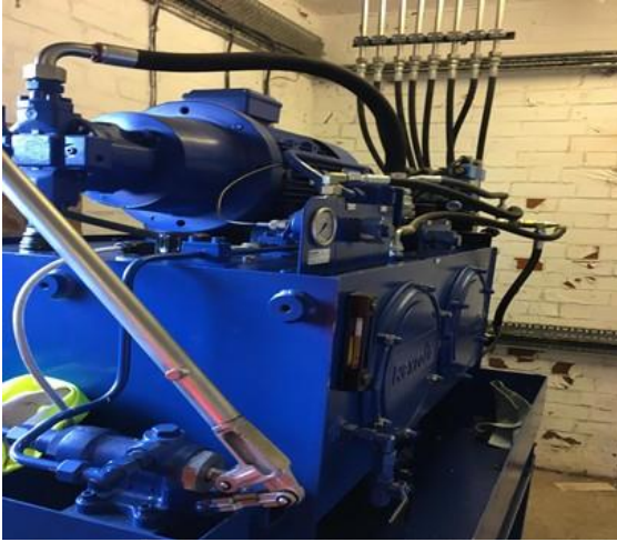
Figure 41: Emergency sluices HPU
