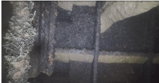
Figure 15: Corrosion on guides– main sluice gate 3
