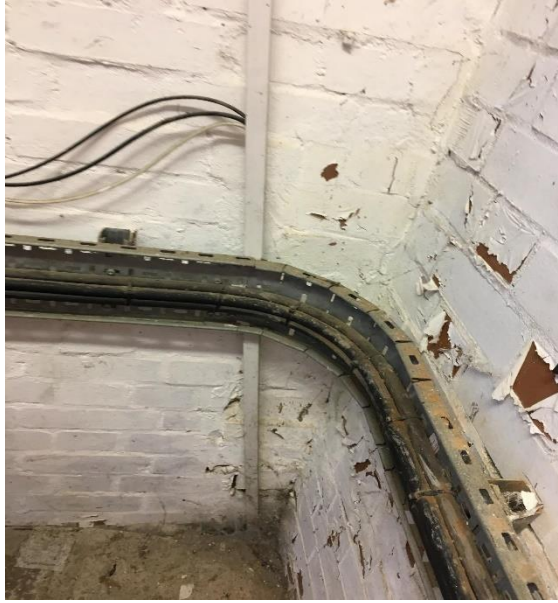
Figure 48: Unsupported cable trunking
