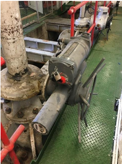
Figure 20: Actuator three – main sluice gate three
