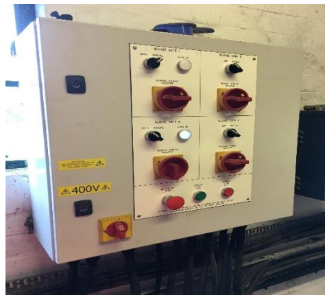
Figure 40: Emergency sluices control panel
