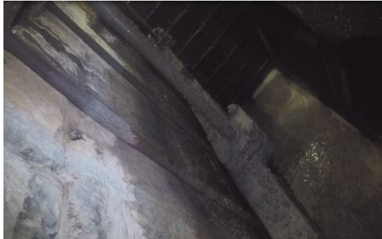
Figure 5: Zebra mussels and corrosion on actuator rising stem base - main sluice gate 1
