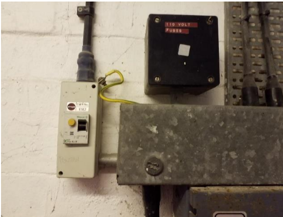
Figure 49: Broken earthing lug
