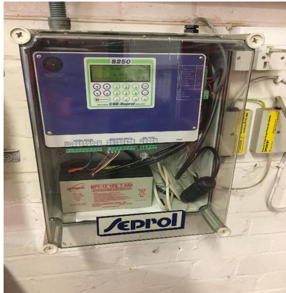
Figure 29: Telemetry outstation
